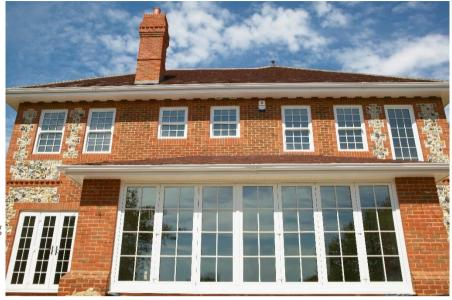
Glazing of up to 62mm thick which allows for triple glazing or acoustic glazing specification. U values are well below the British Regulation targets
